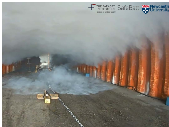
Figure 2: potentially explosive vapour cloud emitted by module in thermal runaway
